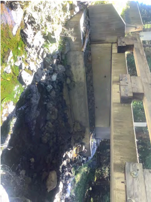
Left Bank Abutment when facing downstream
