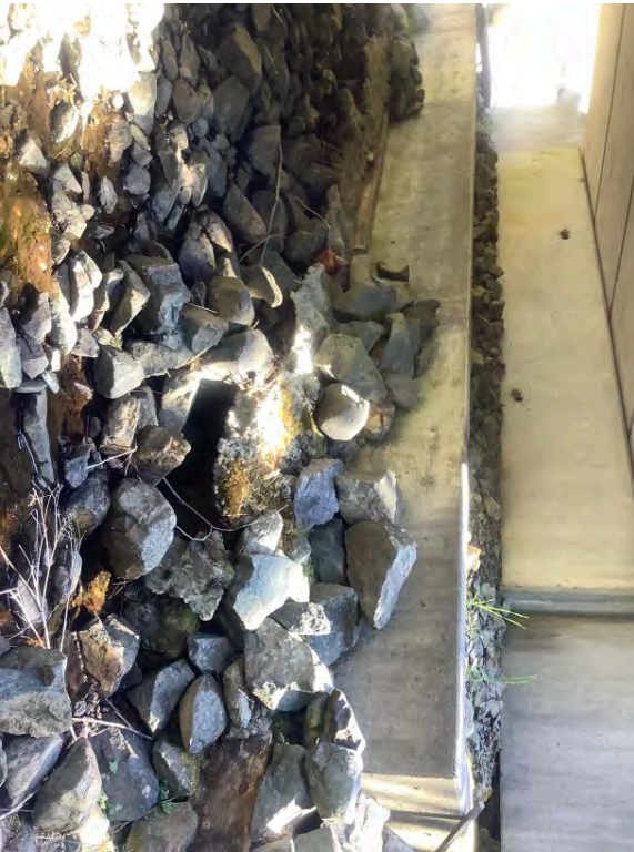
Left Bank Abutment when facing downstream
